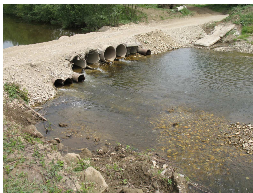
Fig. 1. Hydrotechnic building on Nadrag river (original photo).
